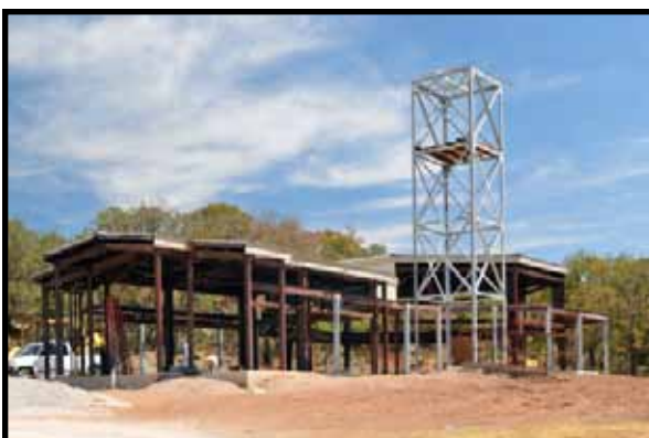
Chapel Construction Progress 9-22
