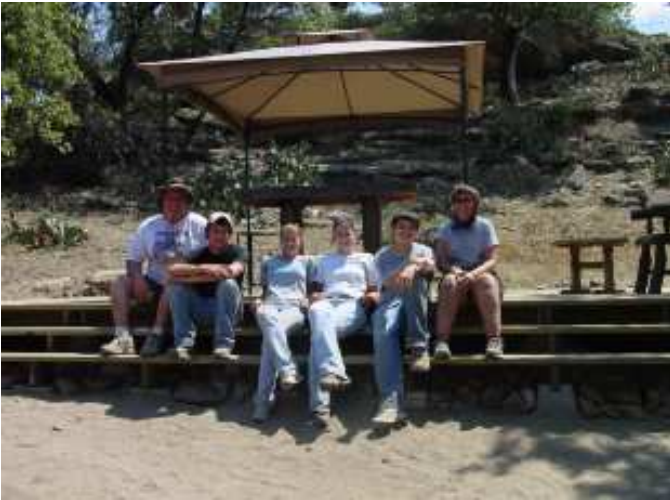
Part of the group worked on the Altar deck for the Chapel
