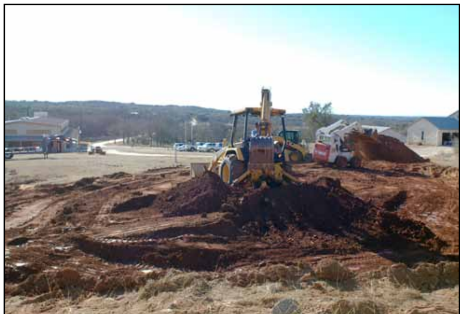
Site prep for the new Chapel
